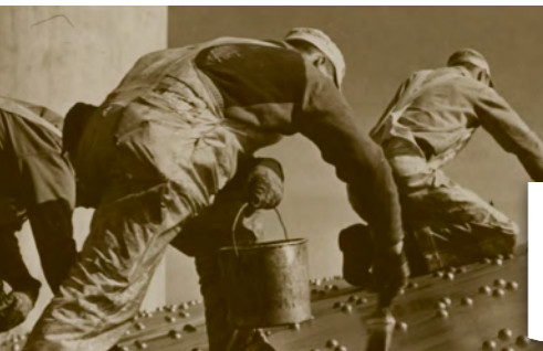
Photo. Construction workers paint a riveted, steel-plated wall on the Hoover Dam spillway. U.S. Bureau of Reclamation, LOC, 1936.
